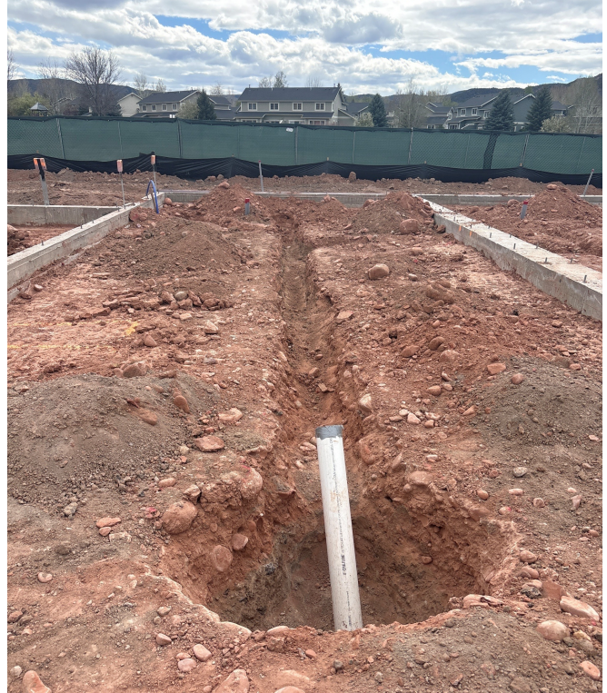
Building A sub slab trenches for plumbing
