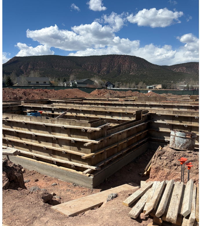
Building A Foundation Walls Formed
