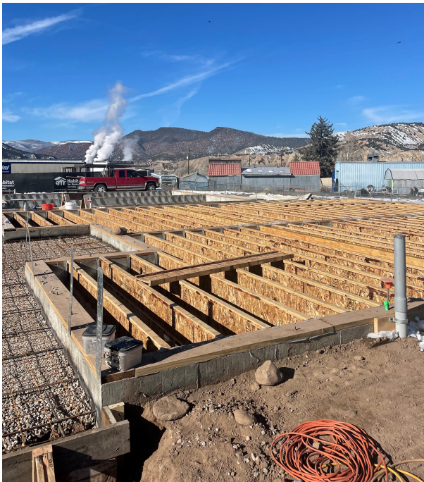
1 st floor joists installed
