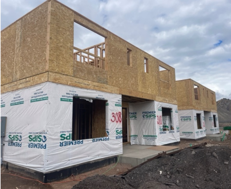
2 nd floor walls complete!
