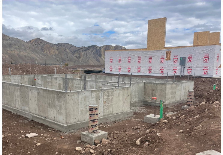
Completed foundations ready for waterproofing and backfill
