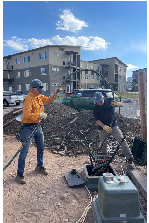
George and Jim help feed wire to each building
