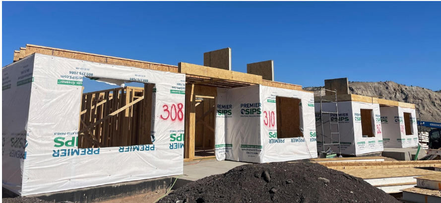
1 st floor SIP panels complete!
