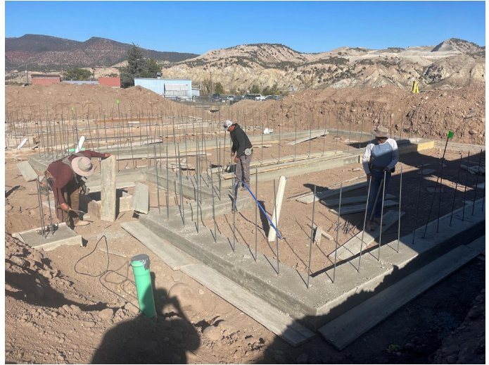
DGO Concrete stripping foundation footer forms
