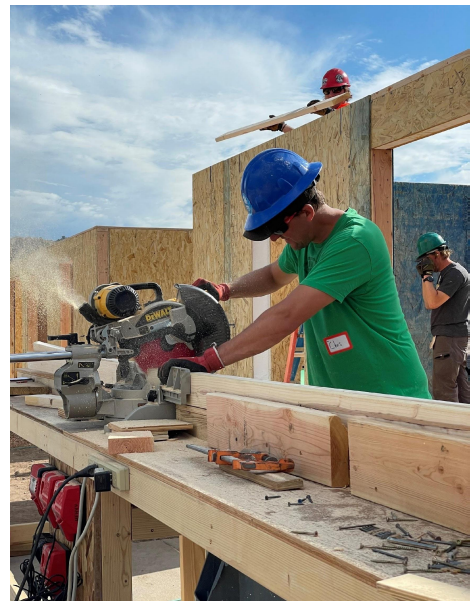
Vail Resorts Employee Chris cuts wall plates
