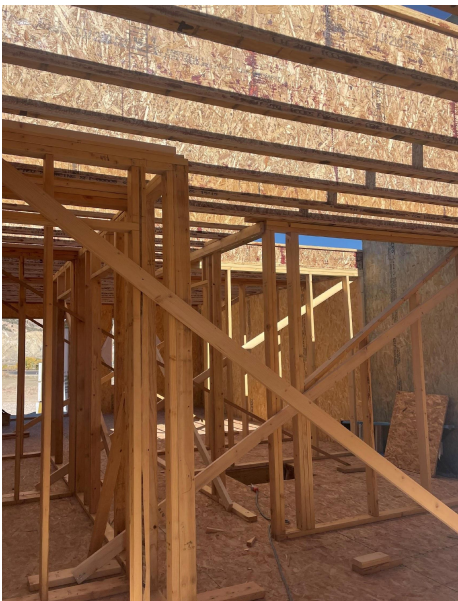
2 nd floor joists installed and ready for subfloor
