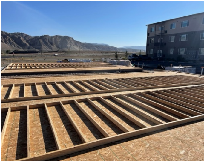
1 st Floor Partywalls framed and ready for raising!
