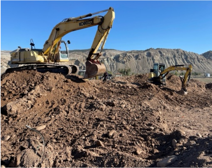
JV Excavation digging new foundations for Phase 11
