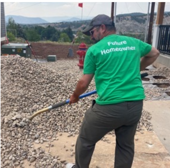
Future Homeowner Mike helping install rock beds!
