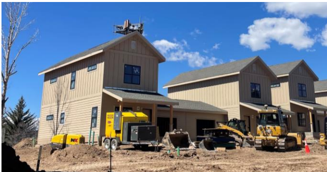
Completed roofing and front porches
