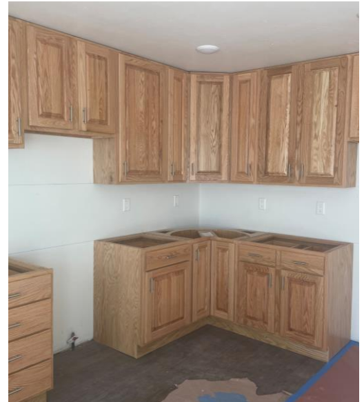
Donna's Kitchen Cabinets Installed
