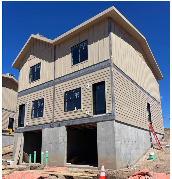
Final modules set in place
