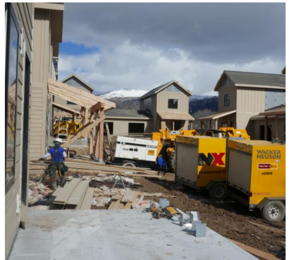
Front Porch Framing
