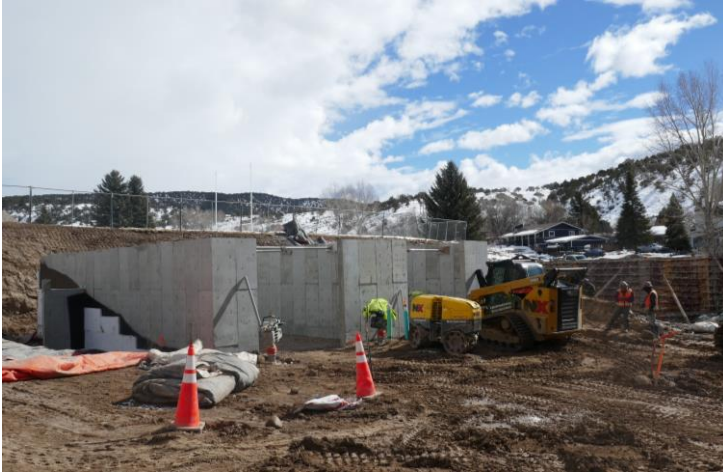
Remaining foundations being poured
