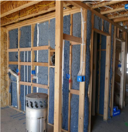
Interior Insulation in Building 5
