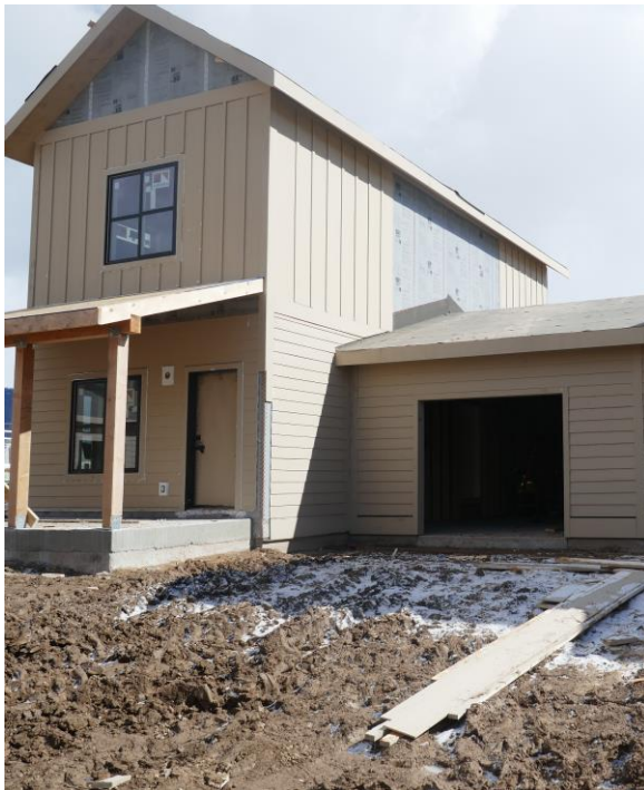
Stick Framed garages completed
