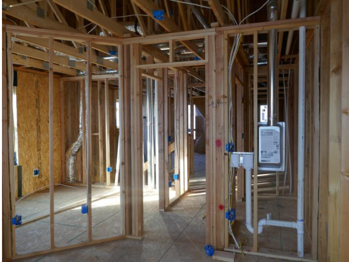
Completed MEP Rough In in Building 5
