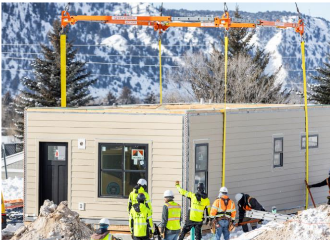
The Set Works team landing the first module
