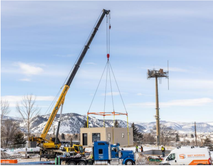
1 st module being set on Adam's Way
